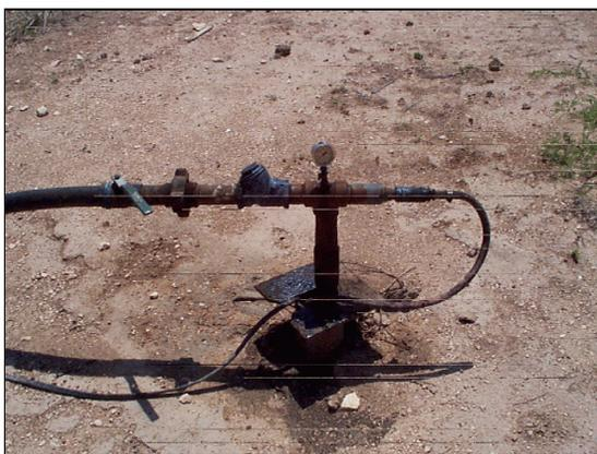
**Figure 1. A wellhead for an electrical submersible pump with a pressure gauge, check valve, union, ball valve, and a hose for checking production.**
