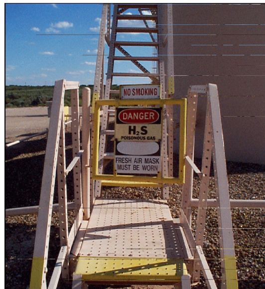
Figure 3. Where \text{H}_2\text{S} gas is present, sour corrosion is likely and breathing apparatus is required.
